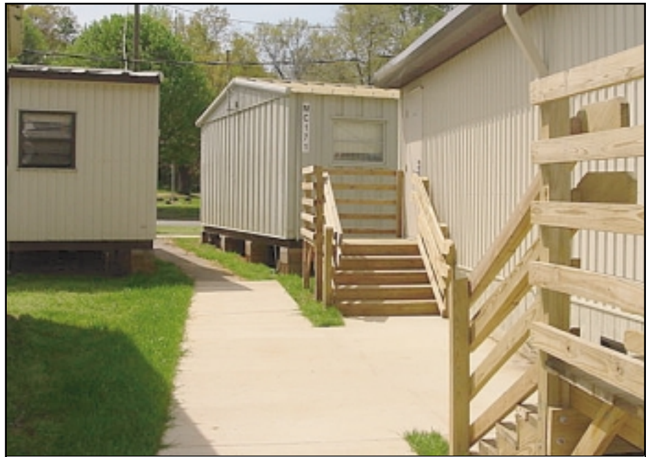
Mobile classroom city at Merry Oaks Elementary. The units will stay until the new school is completed in January. Unit at right is bathrooms.
